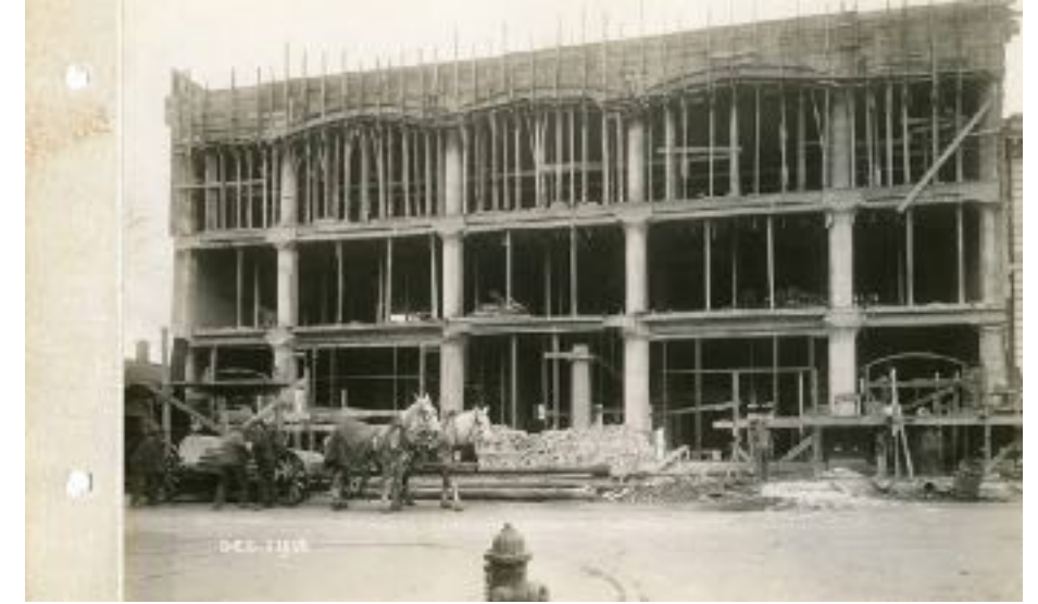
Ford Building construction photo, 1913. Note the horse-drawn wagon transporting a fluted column to be installed at the building's entrance. Photo courtesy Brian McMahon
