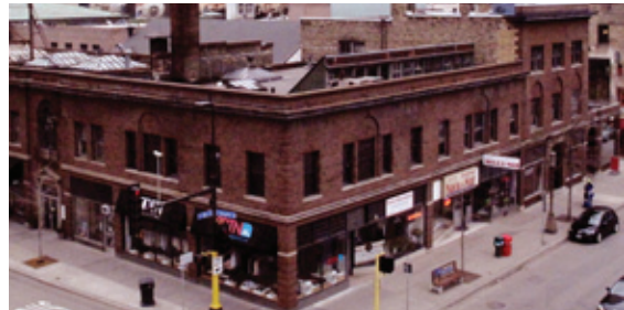
The two-story portion of the Handicraft Guild complex will be demolished. The three-story section at the right will be preserved. Photo courtesy Andrew Dipper.
