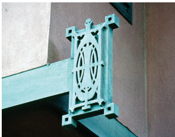
A fret-sawn wood detail on the Hoyt house
