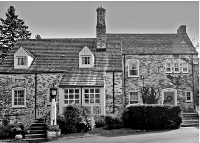
Gainey House, Edwin Lundie, 1945.
