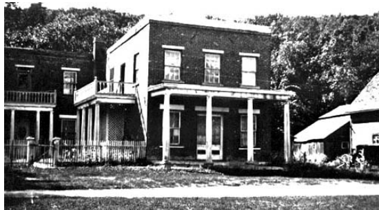
Meighen Store. Oldest surviving building in Historic Forestville, Minnesota, 1923.
